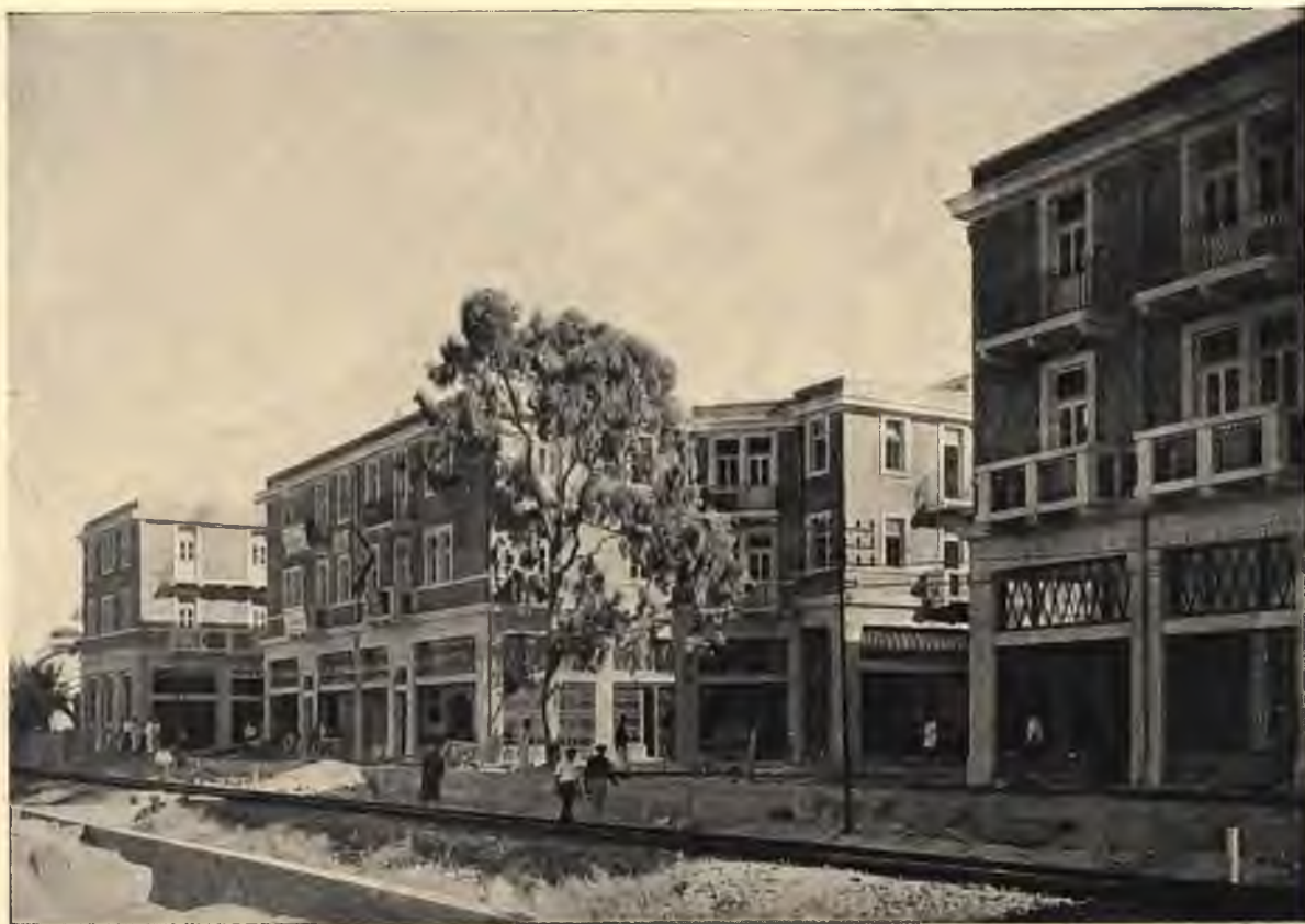
A Section of the New Business Centre, Haifa.
